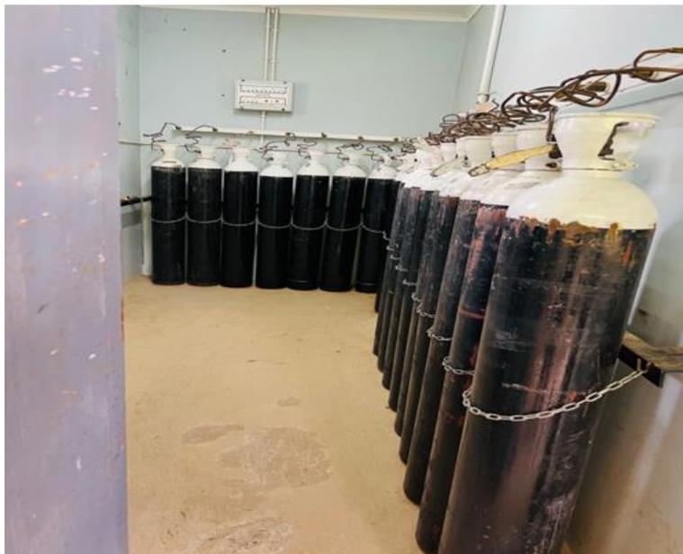
Figure 3: Hlatikulu Government Hospital 2 x 10 Oxygen Cylinder Bank Manifold
